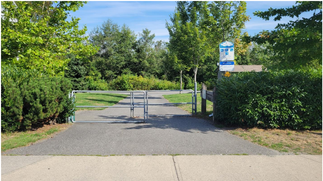
A Fixed Baffle Barrier/Maze Gate (TLR 21) at the entry point of a trail
